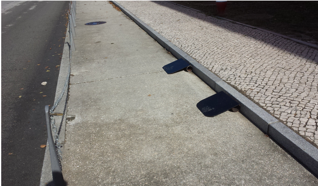
Figure 3.7: Ramp that helps to avoid the collision of the atlascar's chassis with the sidewalk
